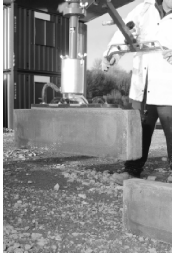
Figure 1 Handling kerbs using a vacuum lifter
